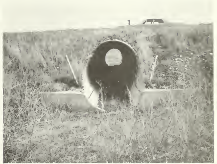
WEST ENTRANCE Note concrete stabilization
